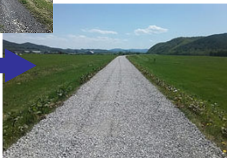
堤防天端の補修
