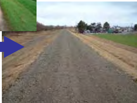
堤防天端の補修
