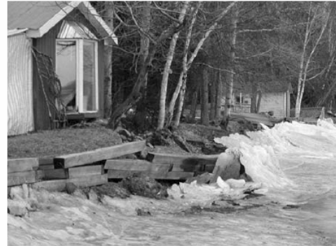
Ice Related Damage on Golden Lakes
