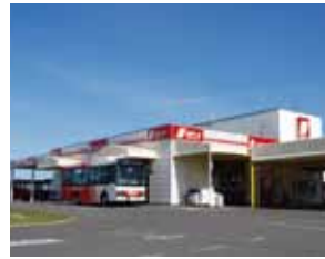
③ Rental car office building
