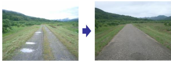
堤防天端の補修
