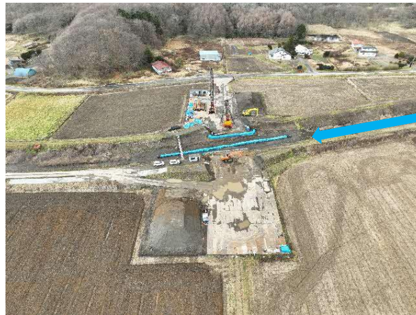
河道掘削 (入鹿別川)橋梁工
