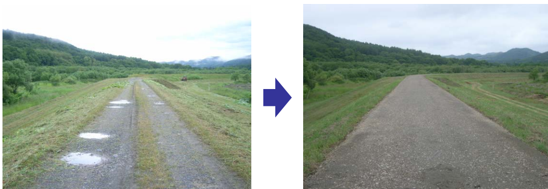
堤防天端の補修
