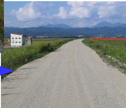
堤防天端の補修
