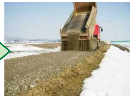
堤防天端の補修
