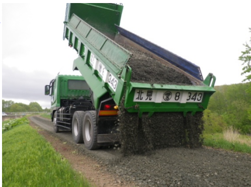
堤防天端の補修
