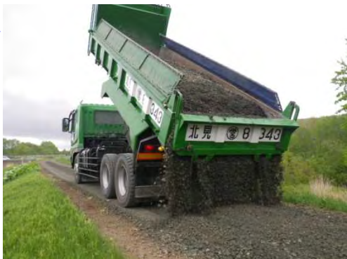
堤防天端の補修
