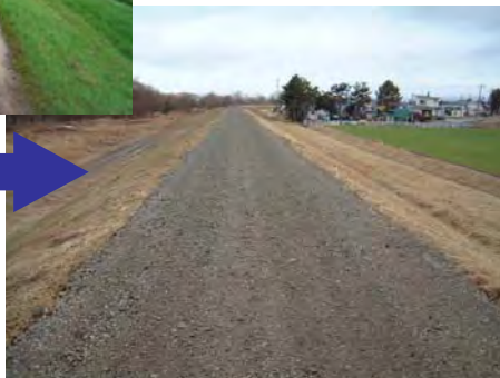
堤防天端の補修
