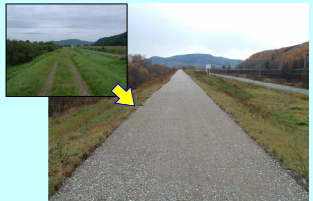
堤防天端の補修
