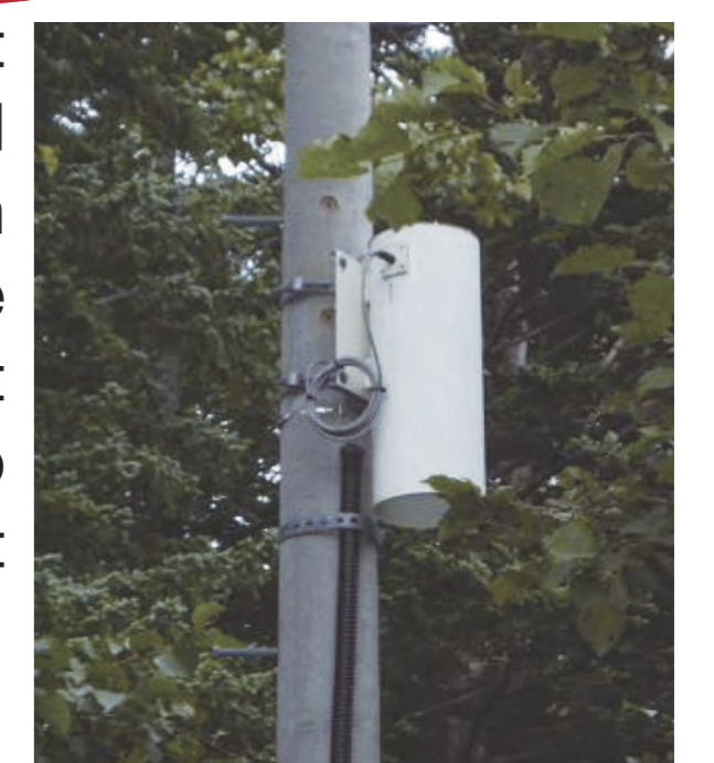
Meters are kept in casing.
