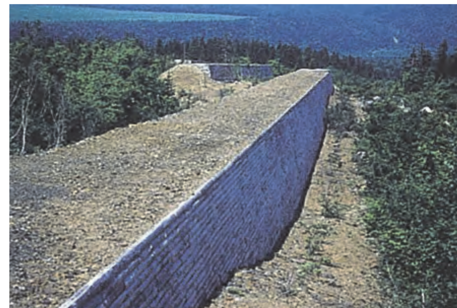
A training dike built on Iousawa, a tributary of the Biei River
