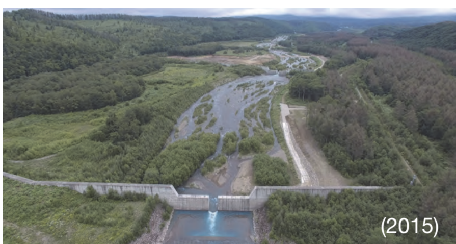
Biei River Sabo Dam No. 8
