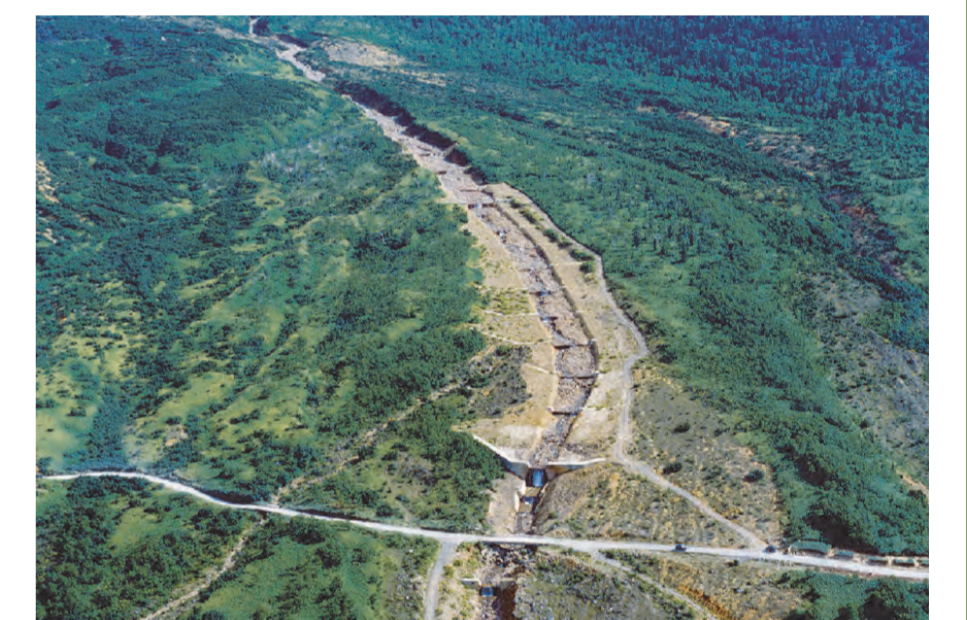
Consolidation work to prevent erosion upstream on the Furano River Photo courtesy of Asahikawa Civil Engineering Office
