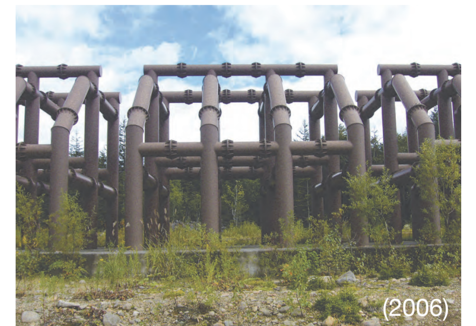
Furano River Sabo Dam (permeable type) No. 2 *Asahikawa Construction Management Division
