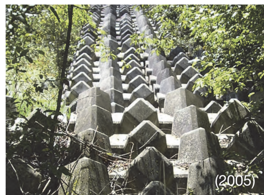
Furano River Block Dam No. 2 is constructed of multiple stacked blocks
