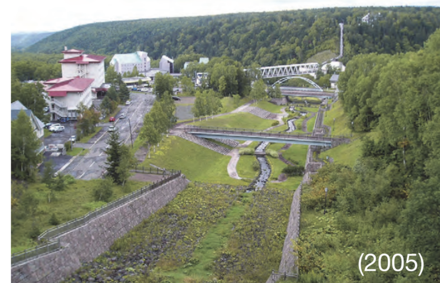
The Tokachidake Channel Works constructed at Shirogane Hot Springs
