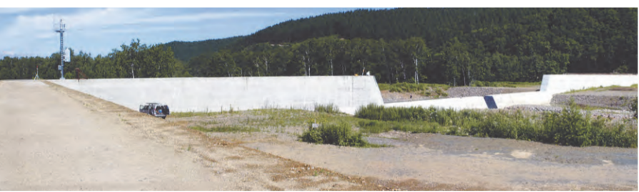
Biei River Sabo Dam No. 5
