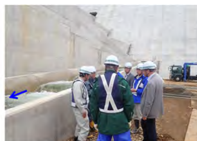
(6/18階段式魚道)流況確認
