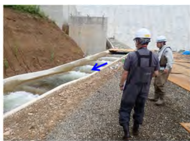
(7/10階段式魚道)流況確認
