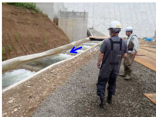
(7/10階段式魚道)流況確認
