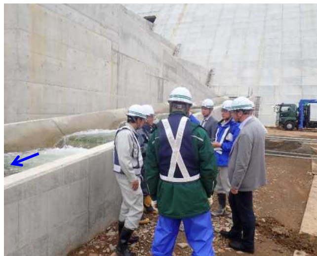
(6/18階段式魚道)流況確認
