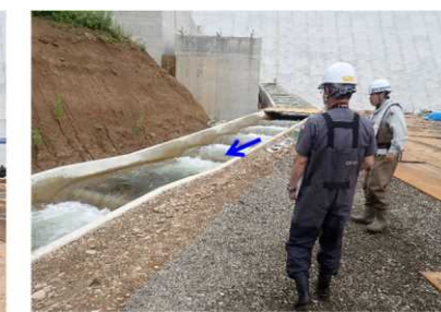
(7/10階段式魚道)流況確認
