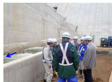
(6/18階段式魚道)流況確認
