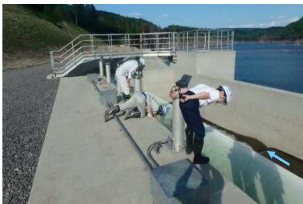
(6/3堤体上流余水) 流況確認
