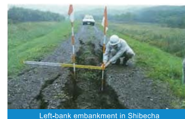
Damage from the Hokkaido Toho-Oki Earthquake in October 1994
