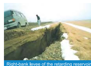
Damage caused by the Kushiro Oki Earthquake in January 1993
