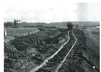
The filling of the embankment
