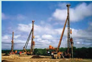
Foundation reinforcement: foundation treated with the sand compaction pile method
