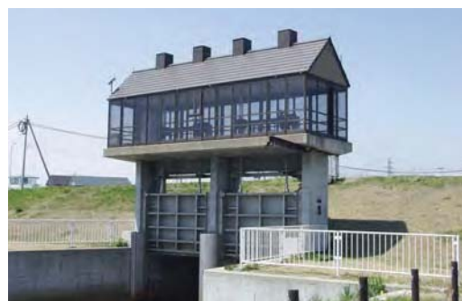
Showa Sluice Way (remote/automatic control)
