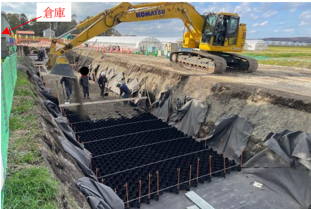
写真-4 ③下段中詰材充填
