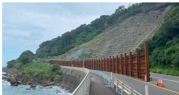
(a) 仮設防護柵
