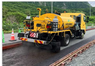
写真-7 As 乳剤の施工
