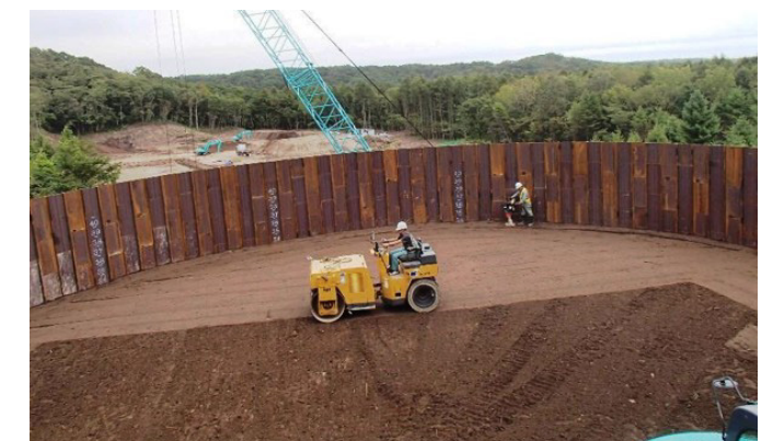
[3] Soil is placed inside the cells.
