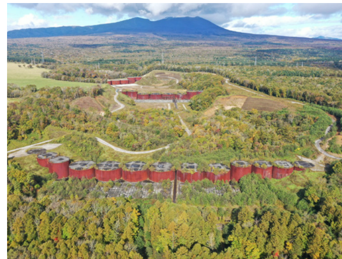
Construction Progress of the Steel Cell-Type Sabo Dam on the Oboppu River
