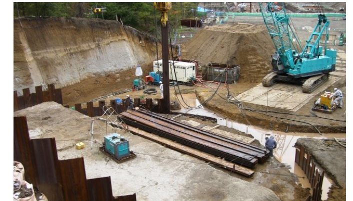
[1] First, long steel sheet piles are first driven into the ground until they reach the firm bearing layer (foundation ground).
