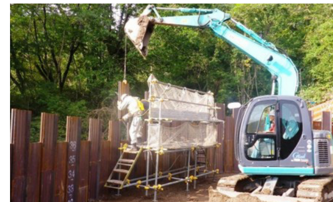
[2] Shorter steel sheet piles are then added to build the steel cell.
