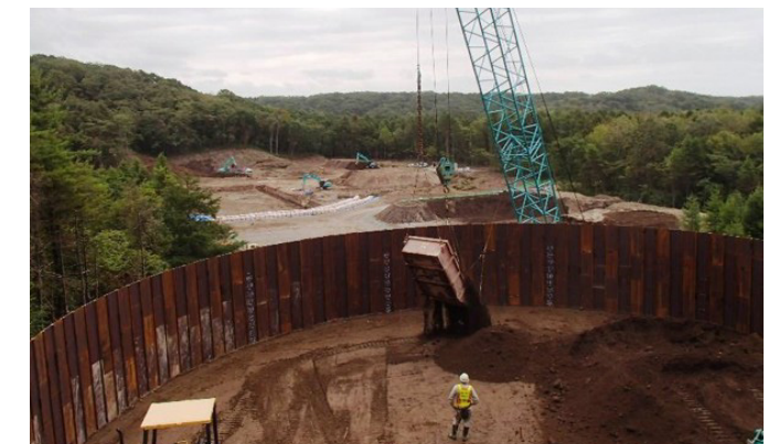
[3] Soil is placed inside the cells.
