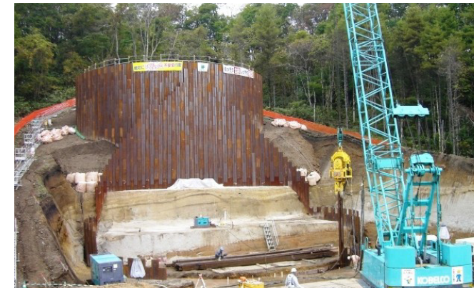
[1] First, long steel sheet piles are first driven into the ground until they reach the firm bearing layer (foundation ground).
