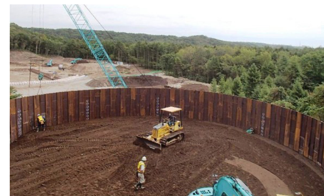
[4] The placed soil is spread evenly and compacted.
