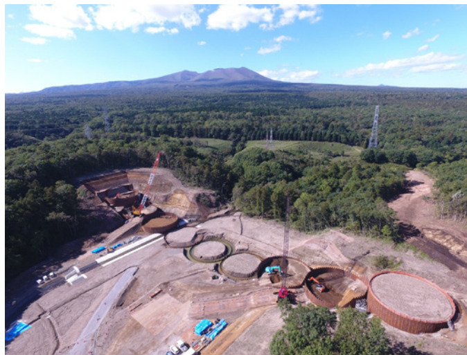
Construction of a Steel Cell-Type Sabo Dam
