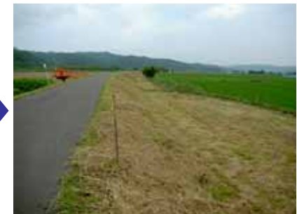
堤防天端の補修
