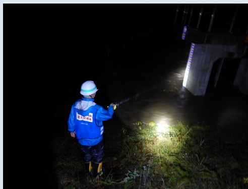
構造物箇所の点検
