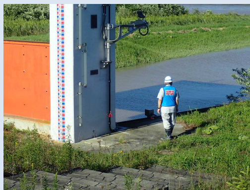
構造物箇所の点検
