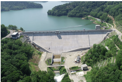
Shin katsurazawa dam
