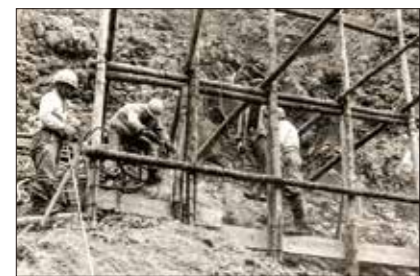
Mortar spraying on the dam body (1969)
