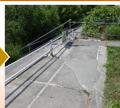
護岸段差補修(豊平川左岸KP15.2)
