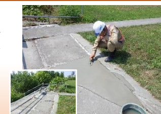
護岸段差補修(豊平川左岸KP15.2)
