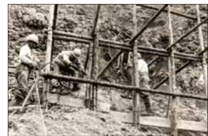
Mortar spraying on the dam body (1969)
