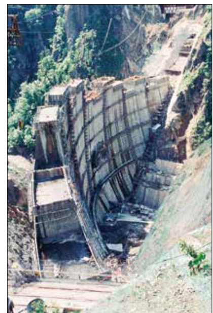
Dam concrete placement (1971)
