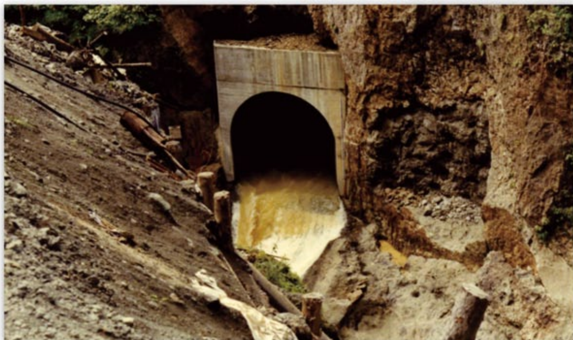
Water flow in the temporary drainage tunnel
