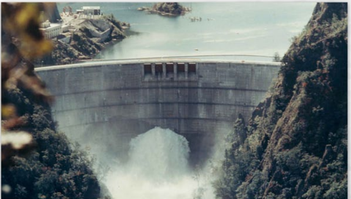
Discharge of water after test filling
