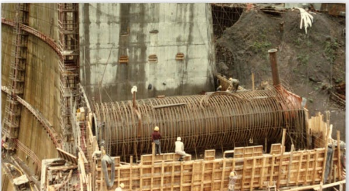
Bar arrangement of the discharge pipe
