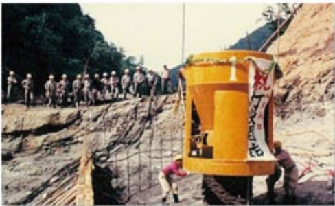
Start of placement using buckets on August 6, 1969
