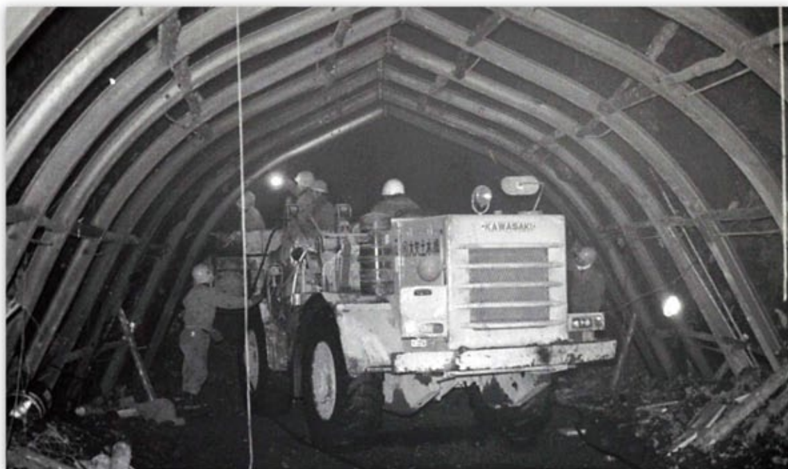
Excavation of the temporary drainage tunnel
