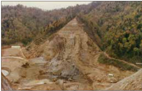
Riverbed foundation excavation (1981)
