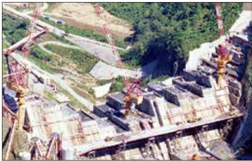
Dam concrete placement (1985)
