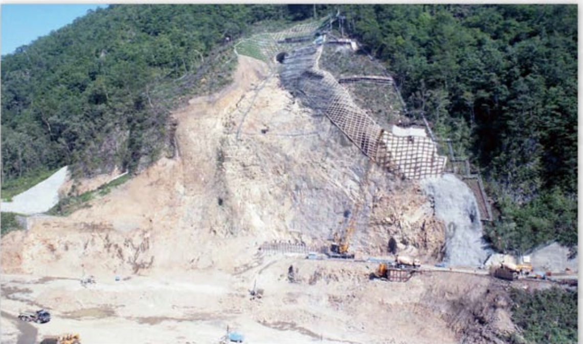
Foundation excavation on the left bank in 1981
